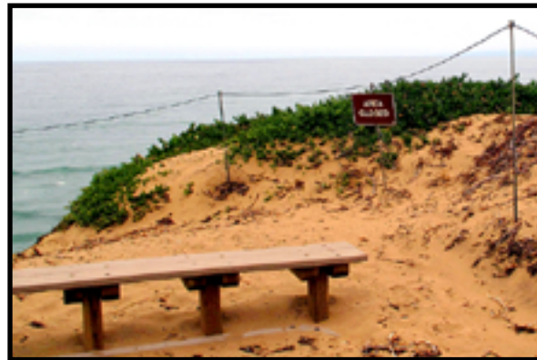
Figure 24. Erosion is a public safety and maintenance concern
